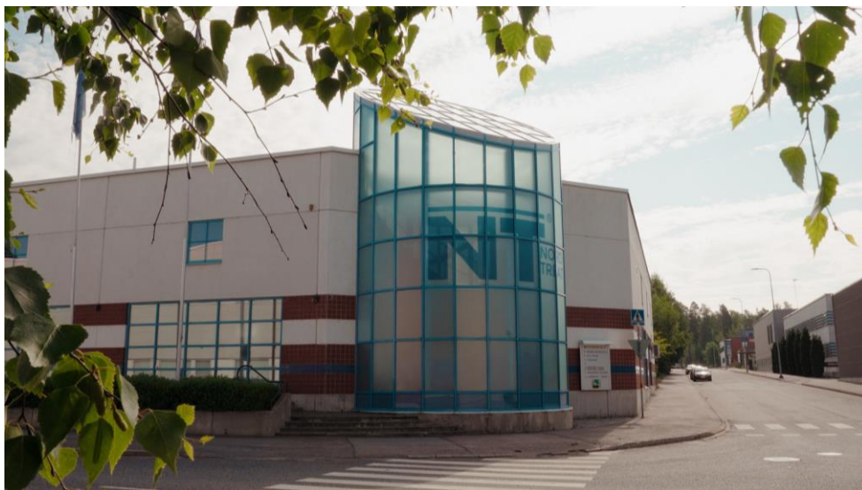
NORDTREAT site in Finland Copyright: NORDTREAT
