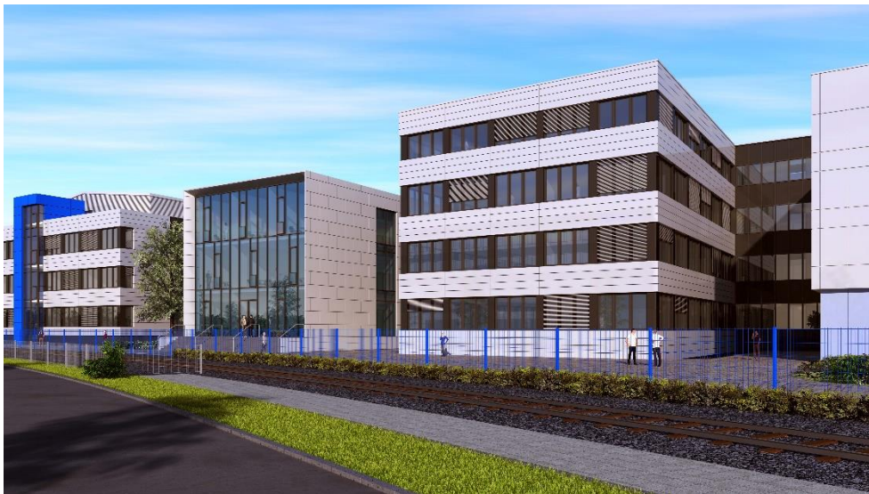
A first drawing shows the " slim part" of the new innovation and seminar complex (on the right) at BYK in Wesel.
